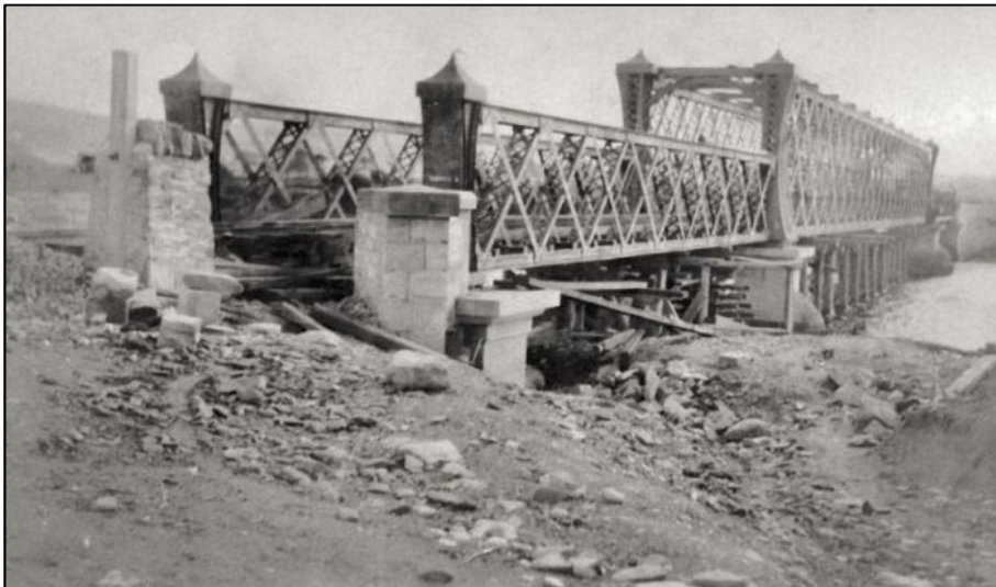
Plate 4: Historic photograph showing the construction of the Lifford Railway Bridge in c. 1909 (source: http://www.sepiatown.com/814657-Strabane-Railway-Station ).
