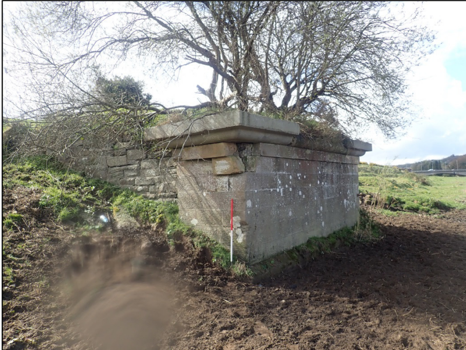
Plate 6: South-facing view of the remains of the masonry railway abutment located on northeast side of the River Foyle (1m scale).
